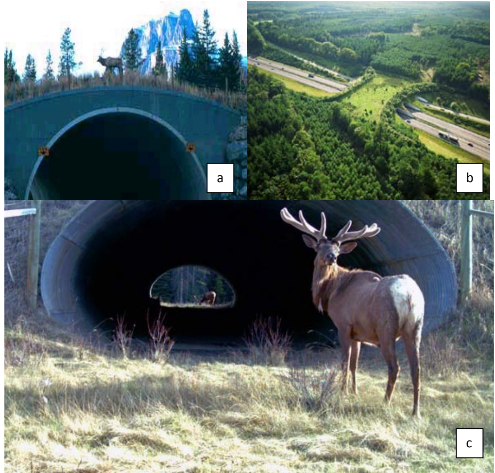
Fig 7.4: Construction of Animal Overpasses (a & b) and underpasses (c) for avoiding road-kills Source: b. http://ecodemica.blogspot.in/2011/01/wildlife-bridge-or-ecoduct.html
